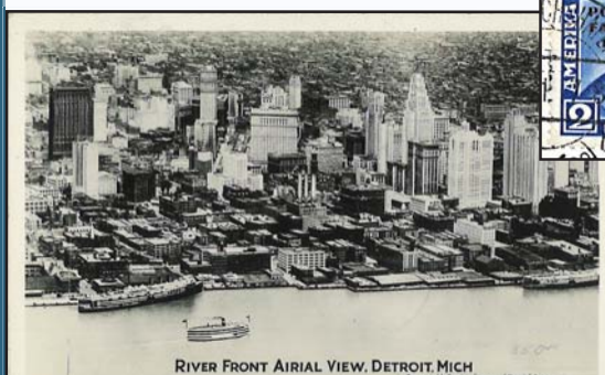
RIVER FRONT AERIAL VIEW, DETROIT, MICH.
